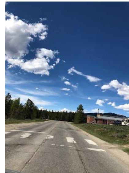
Crosswalk connecting to Aquatic Center and park
