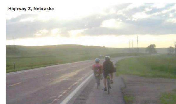
Paved shoulder with rumble strip
