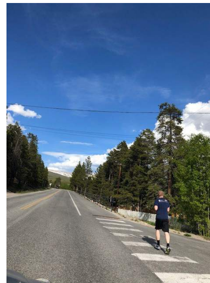
Paved shoulder and crosswalk
