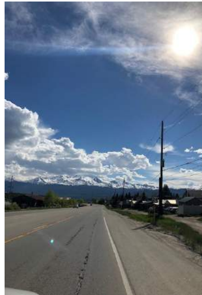
Bike lane turns into paved shoulder and drops off
