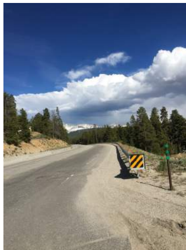
US 24 West shoulder towards Leadville
