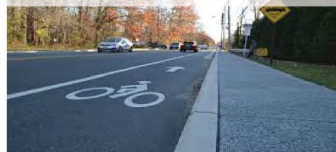
Bike Lane and Sidewalk
